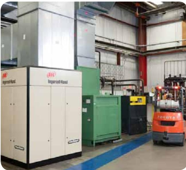
*These industrial-sized air compressors at the Ball DeForest plant see far less use as compressed air is replaced with lower-cost blowers in several applications in the manufacturing process.*
